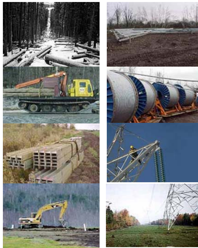
Figure 5-2 –Stages in the process of building a new OHL [205].
