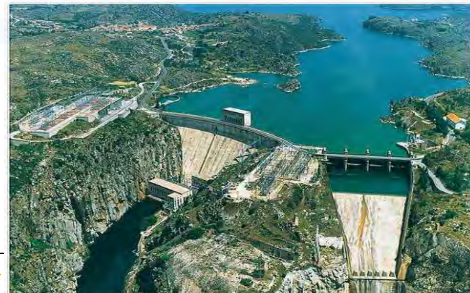
Ricobayo hydroelectric power plant
