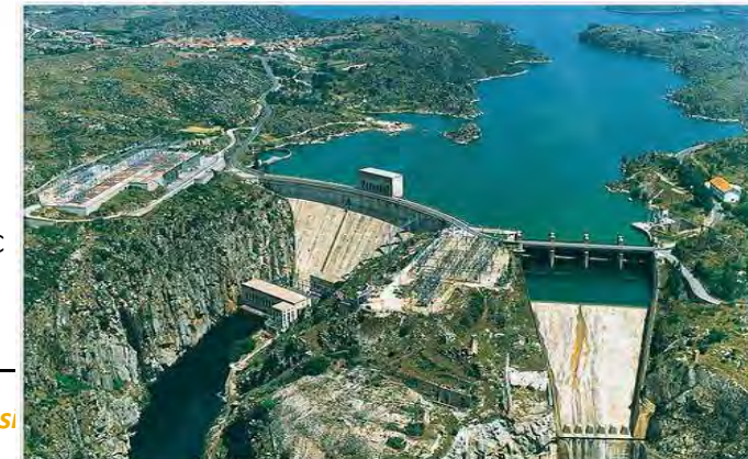
Ricobayo hydroelectric power plant
